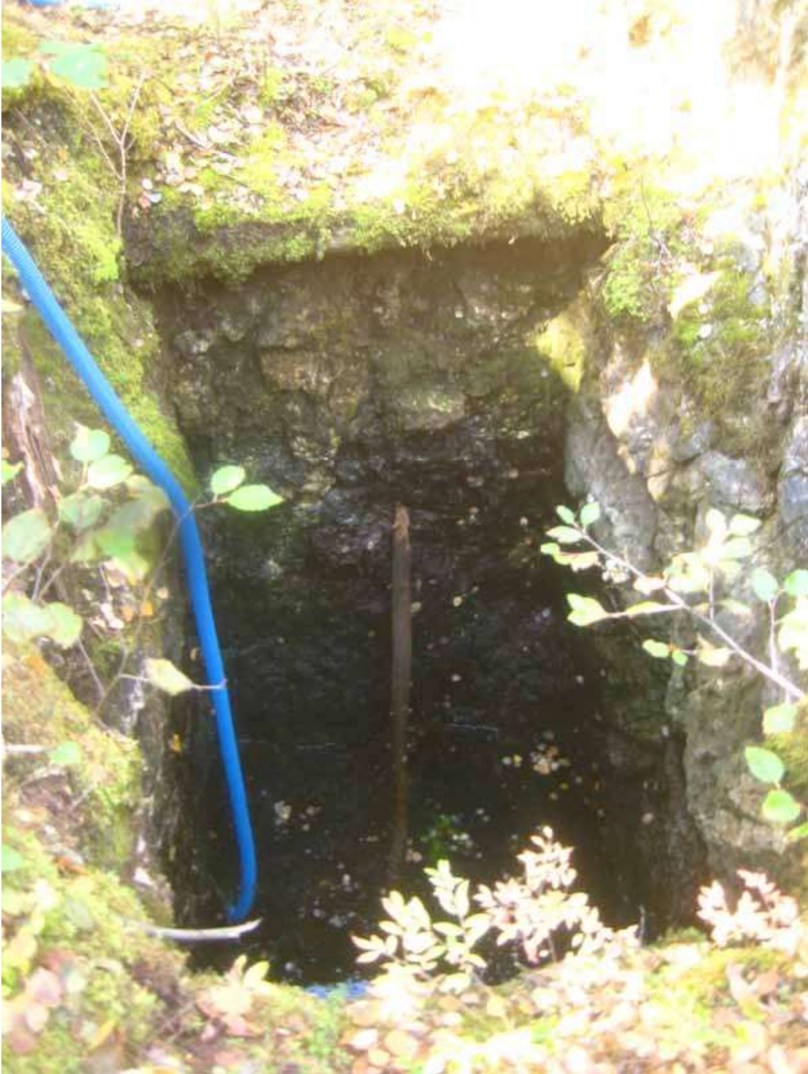
Photo 3. Novack shaft, Deloro Township.
